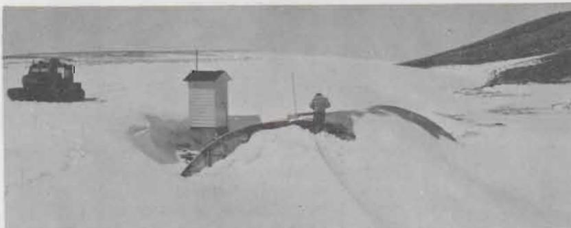
Figure 2.—The arch-covered weir under moderate winter conditions.
