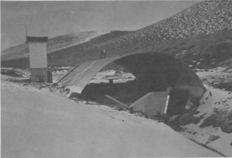
Figure 1.—A sharp-crested weir covered by a multiplate arch. The ends of the arch were later enclosed.
