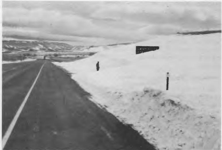
■ SNOW fence really makes a difference. Observe how an informational sign was all but submerged in drifted snow (above) in January, 1971, but stands free and clear in February, 1972. Snow has been trapped by a fence.
