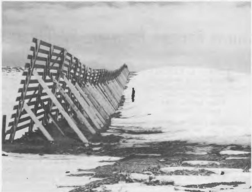
■ WYOMING'S standard-plan snow fence is 12 feet tall and will withstand a 100 mph wind. With treated sills and anchors, its anticipated life is about 25 years. In photo below, effect of a dual-fence system at a former trouble spot is evident.
