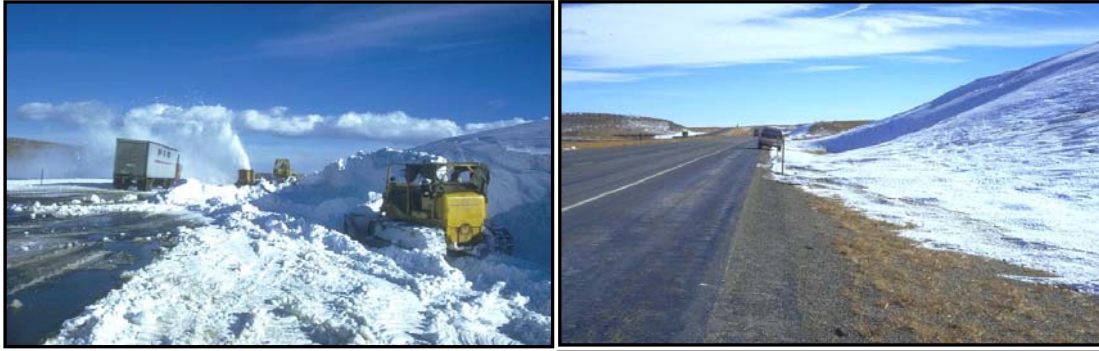
Figure 6. Snow accumulation at RM 274.9 in 1970 before fencing (above) compared with conditions typical of the 35 years since fences have been in place (upper right). The drift formed by the 3.8 m fence was 6 m deep and contained about 80 metric tons of snow per meter of fence length (from Tabler 2003).
