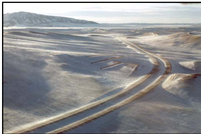
Figure 3. Aerial view of I-80 with blowing snow looking westbound, RM 271 to 268, shows typical topography and vegetation, and one of the first snow fence systems constructed in 1971. Photo Feb. 11, 1972, by R. L. Jairell.
